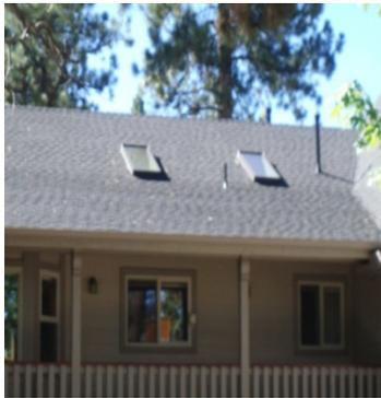
Skylights are another issue that needs to be addressed, specifically plastic skylights. Plastic skylights can melt with radiant heat and/or direct flame impingement. Also, the accumulation of fire brands can and have melted skylights resulting in an opening that allows significant accumulation of fire brands to enter the structure. Once inside, the contents ignite and the structure burns from the inside out.
